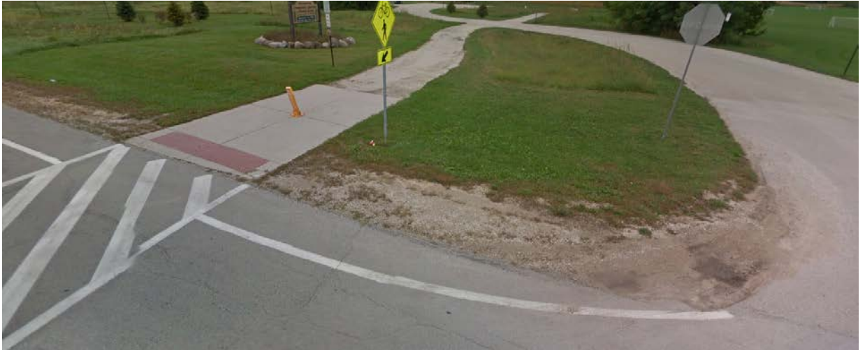
Figure 10 – Existing Southwest Curb Return
