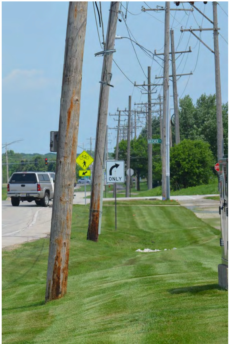
Figure 18 – Utilities on the East Side of Peck Road
