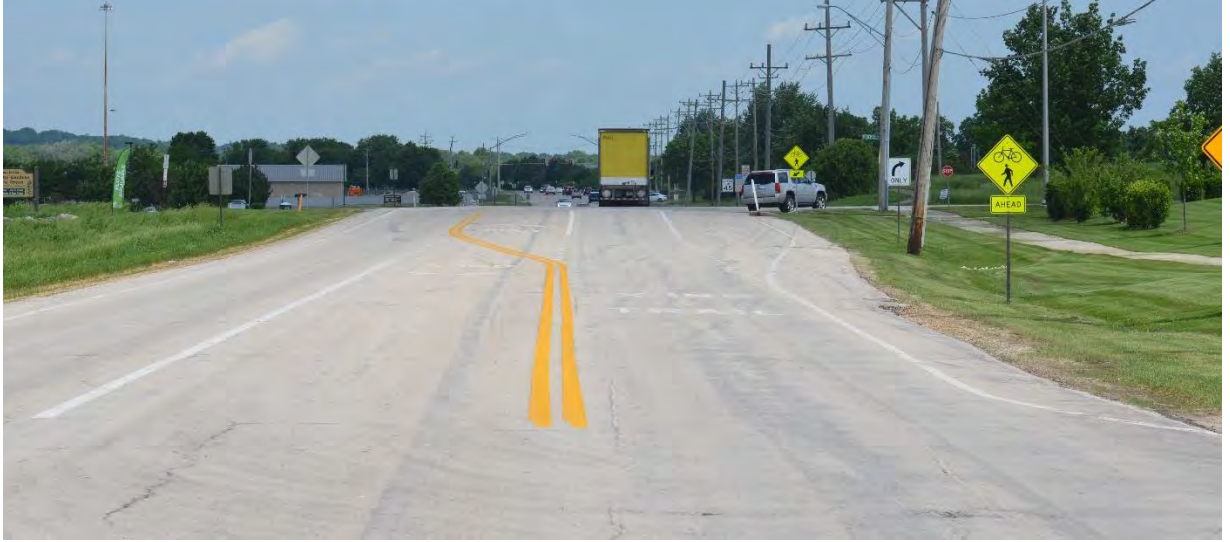
Figure 15– Photo of Vertical Curves south of intersection looking north
