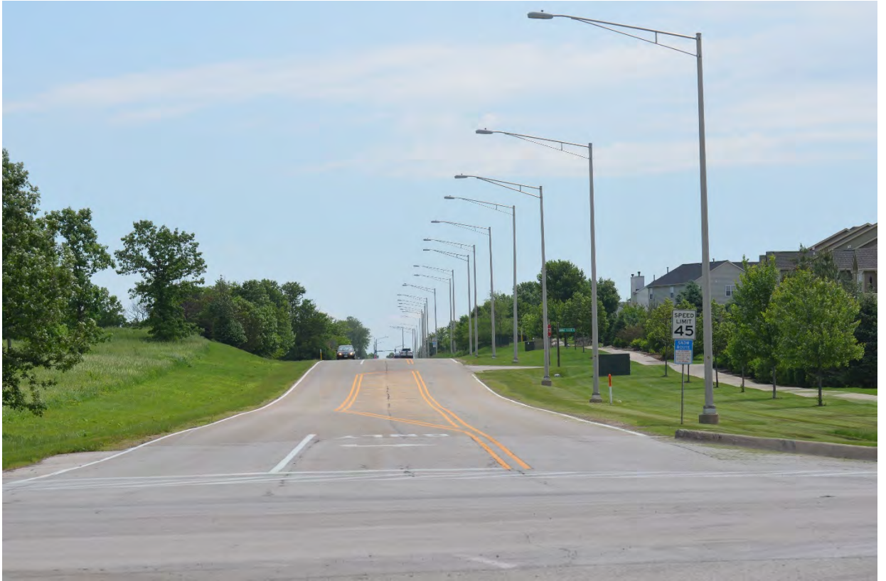
Figure 4 – Photo at intersection looking east at Bricher Road
