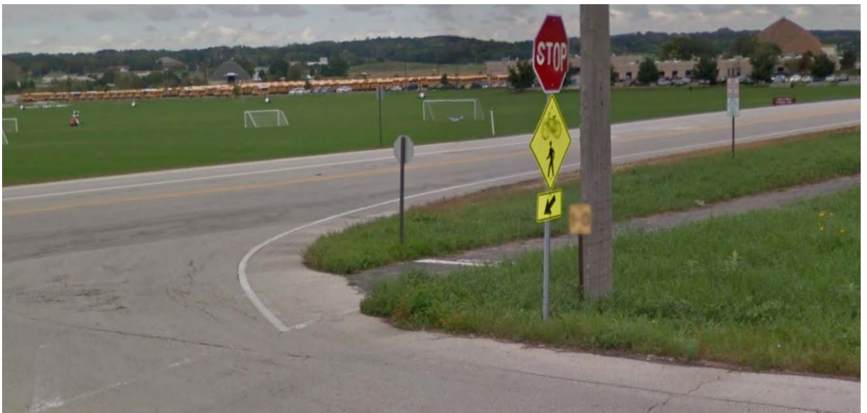
Figure 9 – Existing Northeast Curb Return
